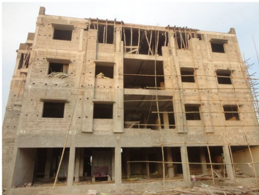
De bouw is in volle gang
